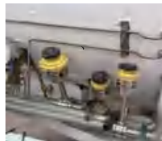
FB V4 Valves used in LNG tanks
